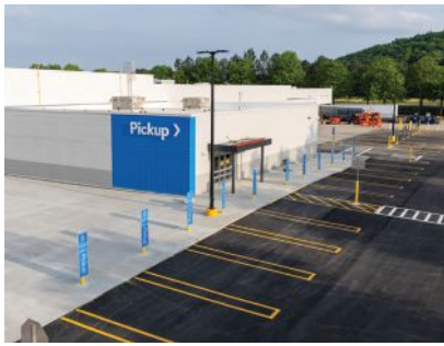
3DCP is safer, faster and cheaper than traditional concrete masonry construction.
